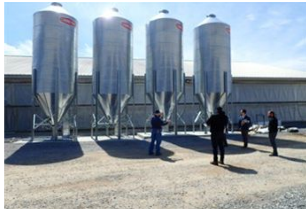
▲ Feed bins installation at the ETREC-Little River Unit freestall barn
